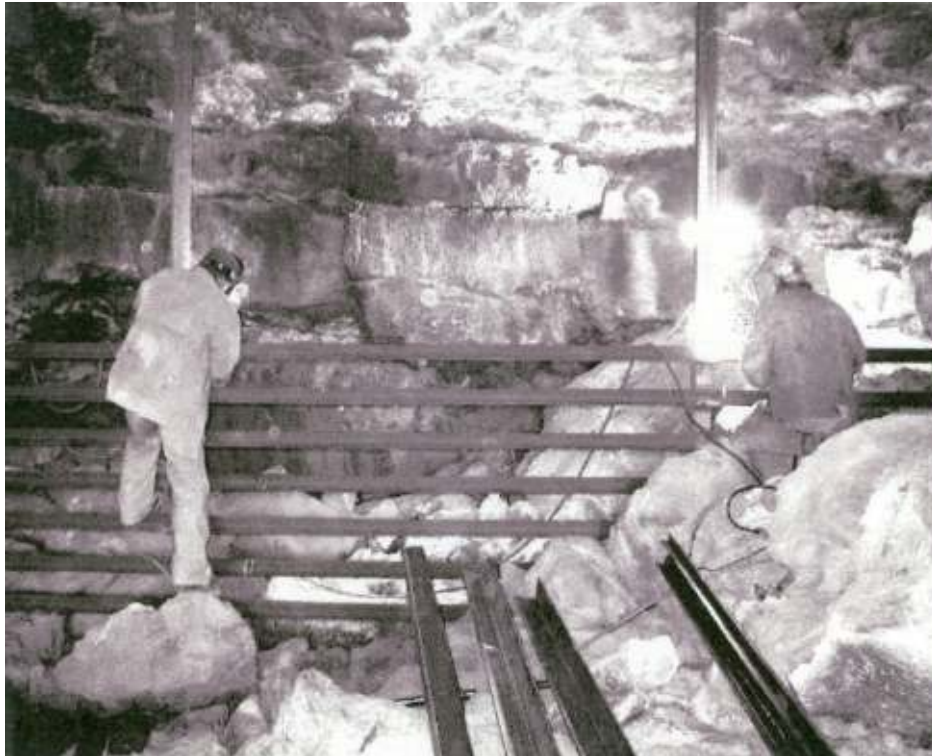
Two welders working simultaneously on the Stookey Ranch Cave gate. 9-00.
