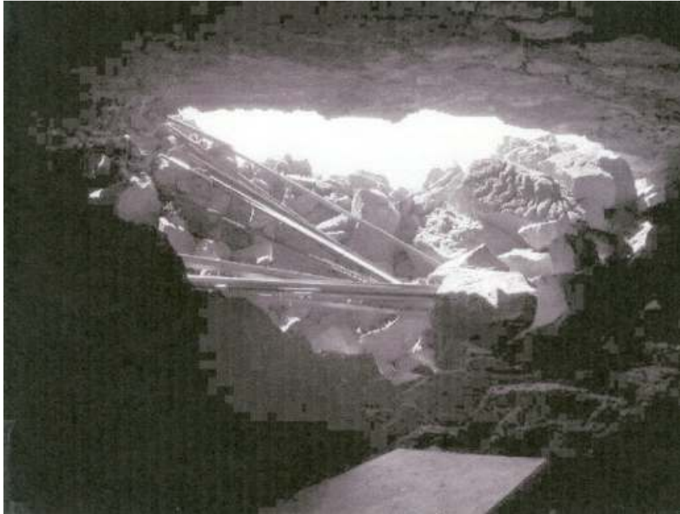
Staging the gate materials at the entrance to Stookey Ranch cave. 9-00.
